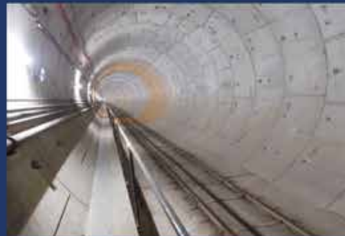
Shield Tunneling Method
